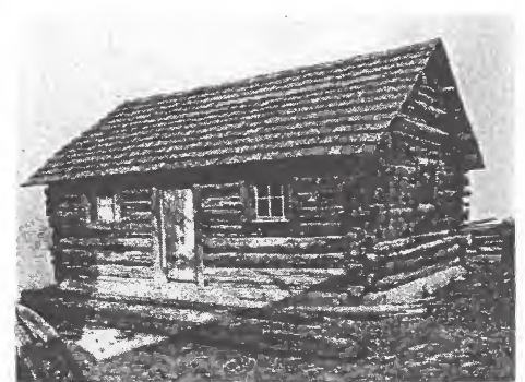
Pony Express Station at Pioneer Village. Old log cabin of Jim Sharp (SUP's Pony Express authority) brought from the Sharp ranch at Woodland, Utah, by the Ute Ranger's Mounted Posse. The enclosure will be authentically furnished inside with extant Pony Express relics.
